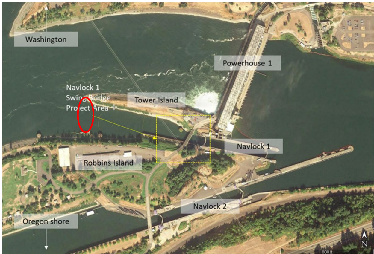
Figure 1 - General site layout for Bonneville Dam Navigation Lock 1 Swing Bridge Replacement. Area circled in red indicates where sea lion traps are operated by other entities.
